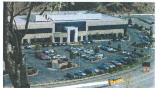
Parking lot, Sierra Point.
